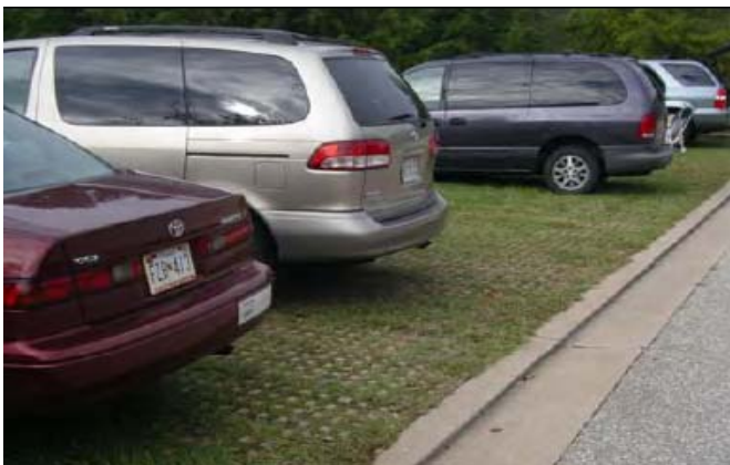
Permeable parking pavers can help reduce impervious coverage. Source: New York State DEC Stormwater Manual, 2009
