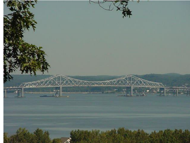
Tappan Zee Bridge
