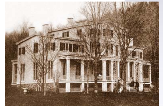
Jacob Sloat House (Harmony Hall), Sloatsburg
