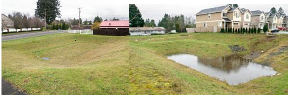
Figure 6. Empty infiltration basin Figure 7. Infiltration basin after storm
