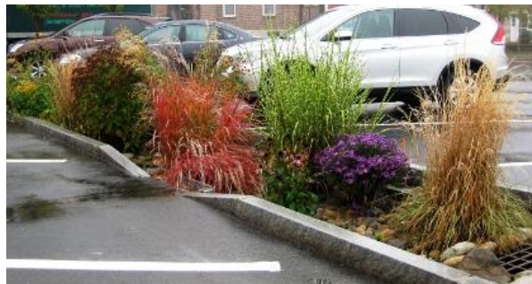
Figure 5. Rain garden implemented in a parking lot
