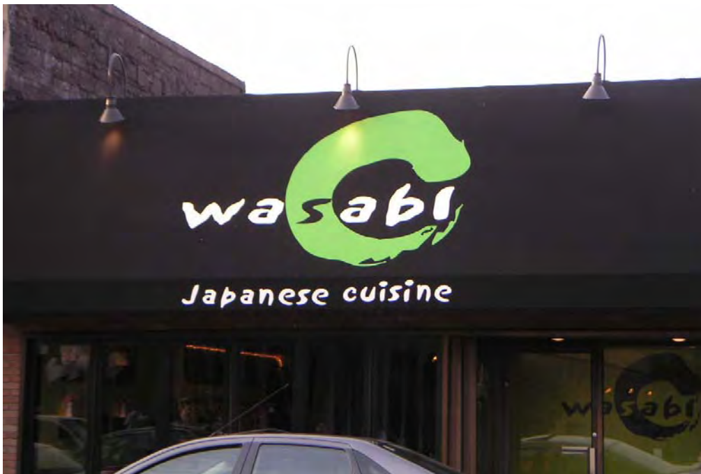
Awning lit by goose neck lighting.
