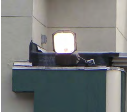
Lights such as this pose a danger to motorists by shining into the roadway.
