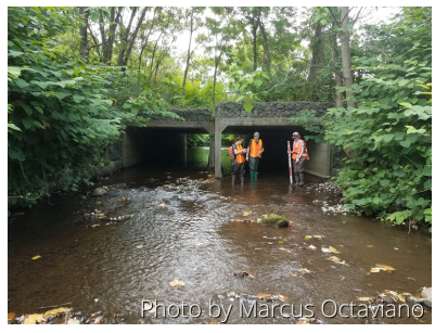
Photo by Marcus Octaviano (Above) Seasonal staff measuring the dimensions of a box culvert
