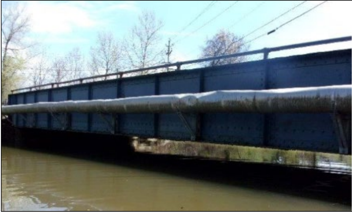
Gagan Road Bridge Elevation Looking Southeast
