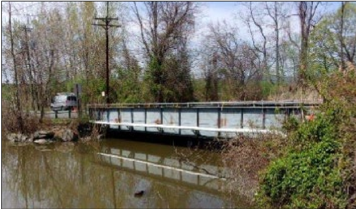
Gagan Road Bridge Elevation Looking Northwest
