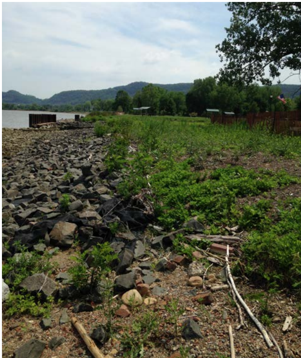
Figure 4. View from northern beach looking to the south. From left to right: displaced rip-rap, wrack line, and transition zone between native planting buffer (not yet planted for this year in early summer 2016). There was some re-grading of this low slope area at the far left where low banks were undercut.
